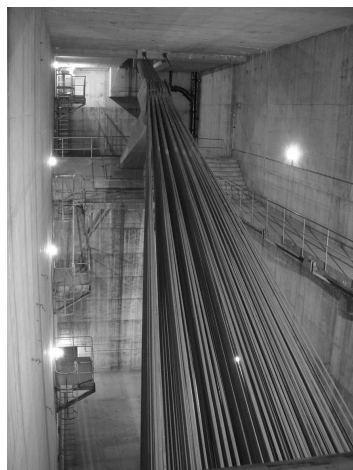
(b) North-west anchorage chamber
